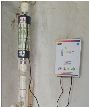
Akshat Tower Pakwan Cross road, Ahmedabad
